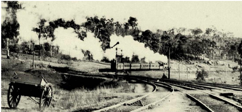
Figure 9 Steam Train leaving Walcha Rd Station in the 1920s xvii
