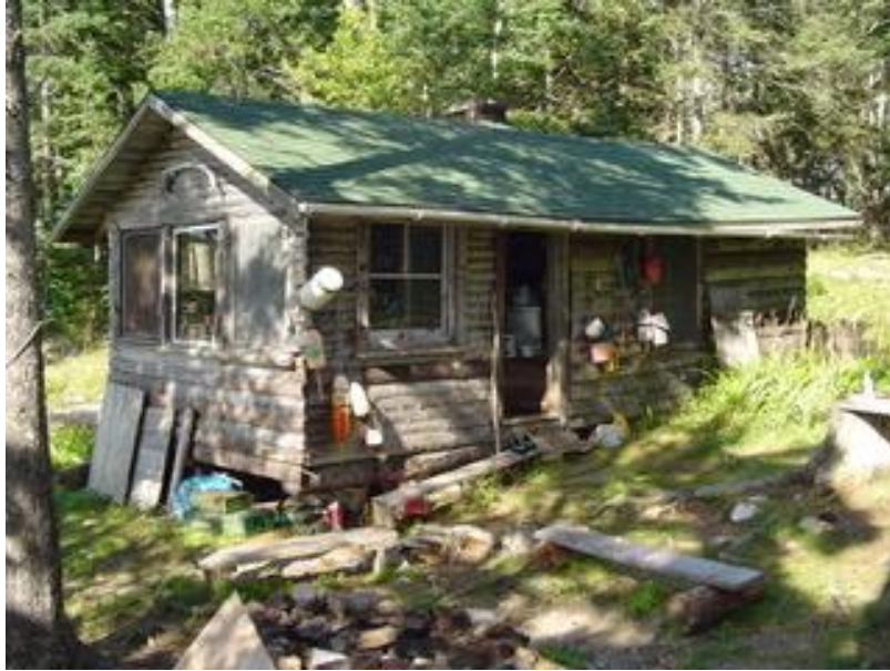
Our cabin in the 1960s, after the roof had been repaired
